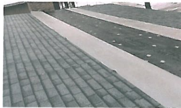
Residence where Rayco installed Shingle-Ply
