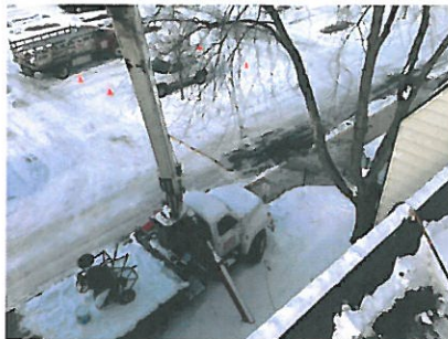
Rayco battled the elements to re-roof Lincoln Place Apartments in Mahtomedi
