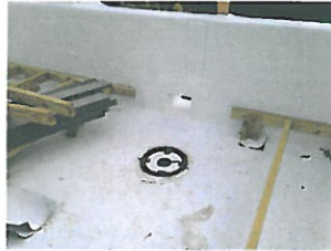
Scupper cut into wall at Colfax Apartments
