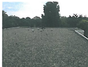
Ballast EPDM roof Rayco installed at 1776 St. Clair Ave
