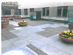
Pavers installed over TPO membrane at Langton Place in Roseville.
