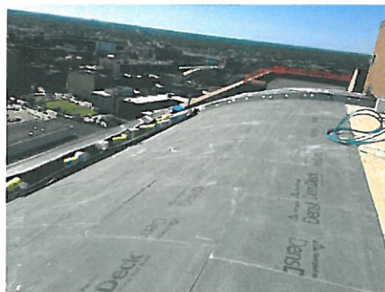
DensDeck® installed at the Churchill Apartments.
